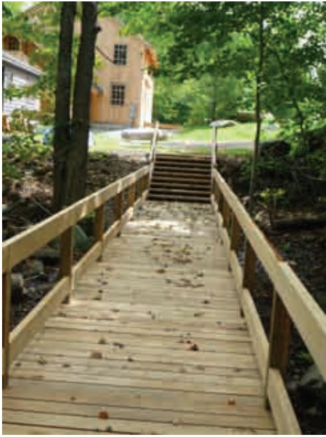
The new bridge safely connects the Resource Center to the Fisher Family Activity Barn.
