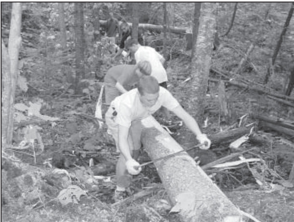
Jimmy Elcock and Pier Pennoyer peel bark from a spruce tree to construct a bog bridge on Mead Trail during session two of Squam Conservation Corps. Photo by Eric Morse.
