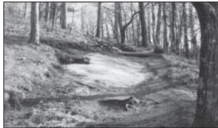
Before... The steep eroded ledge was causing the trail to widen. Photo by Eric Morse.
