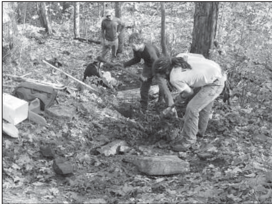
Nelson Bruni and Atticus Doman construct a waterbar and step on the upper section of the Mt. Morgan Trail. Photo by Eric Morse.
